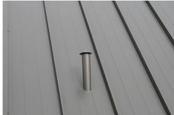
Avoiding the use of long back trays helps achieve an aesthetically attractive solution for penetrations
